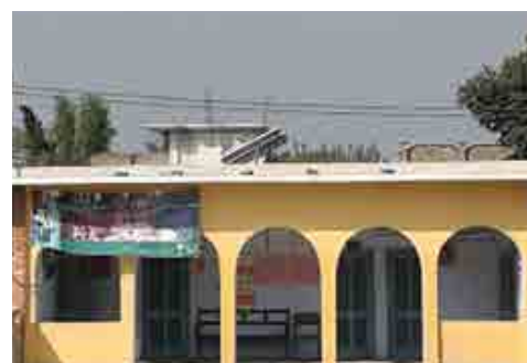
Newly installed solar panel for electricity backup at BHU Khazana Deri, 2017.
