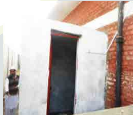
Newly constructed toilet for female patients at BHU Khazana Deri, Mardan, 2017, based CBO-led advocacy
