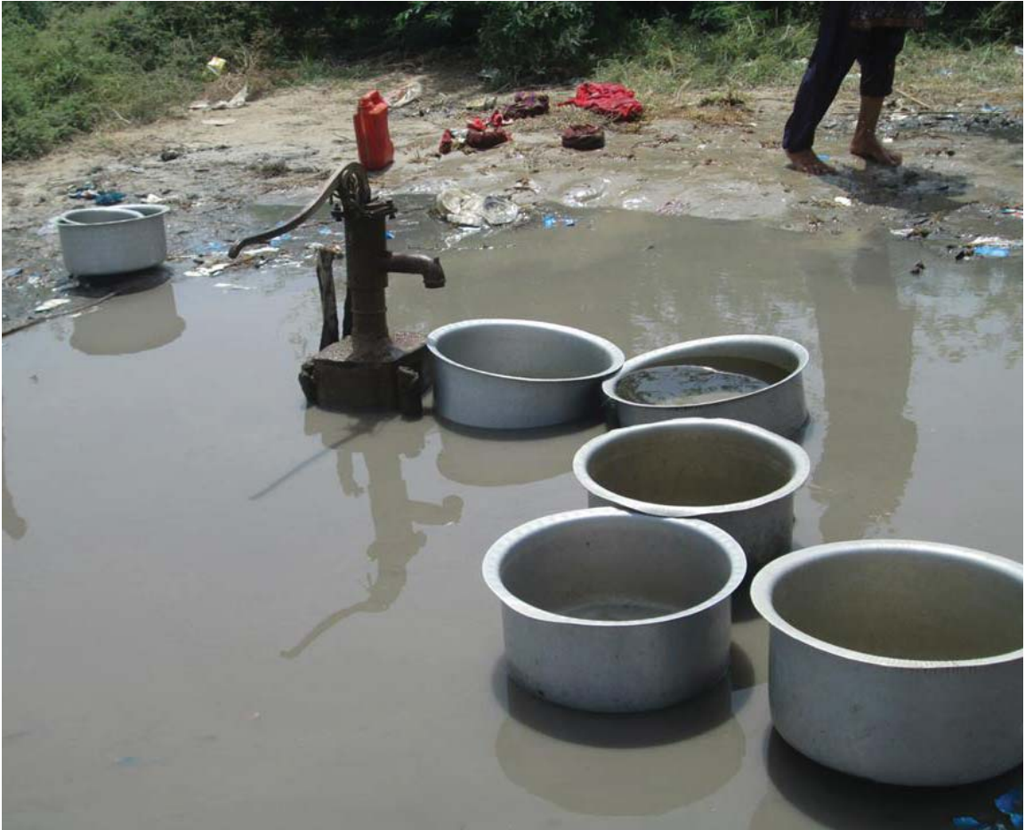
Hand pump at Haji Manjhi Otho Village
